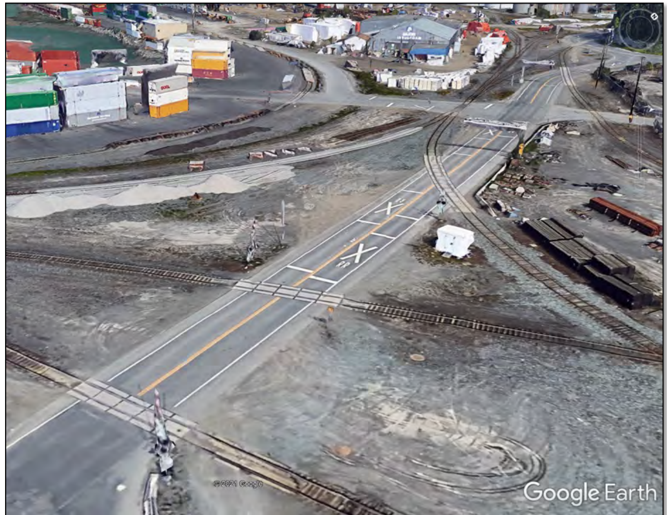
A portion of the study area, which includes five closely spaced railroad crossings.
