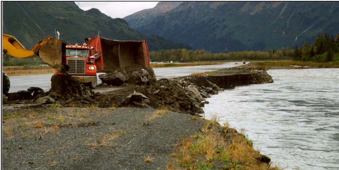
Figure 21: Maintenance and Operations crews doing emergency repairs to end of runway.
