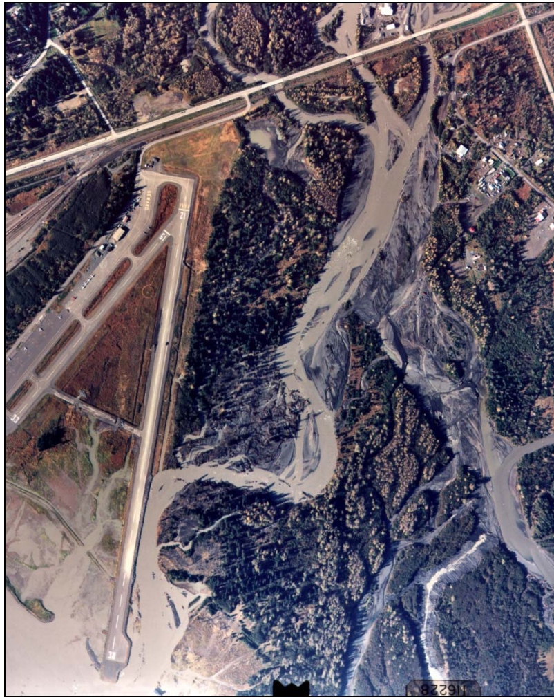
Figure 36: Aerial photograph taken after the October 1995 flood event.
