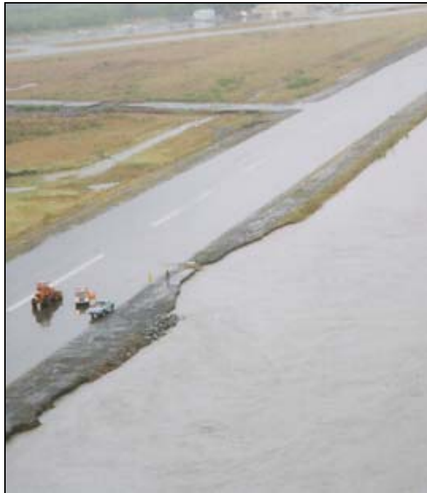
Figure 20: Maintenance and Operations crews doing emergency repairs to end of runway.
