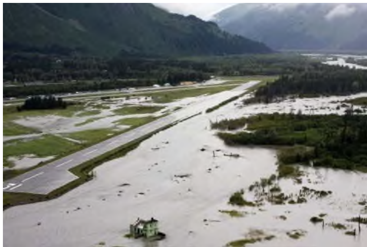
Resurrection River in flood stage overtops main runway of Seward airport. Photo courtesy of Seward/Bear Creek Flood Service Area.
