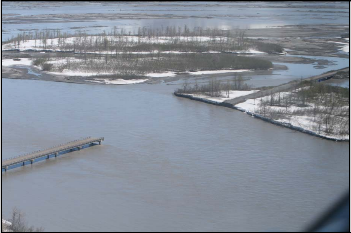
Figure 2 – Road breach east side of Bridge 339 June 9, 2013
