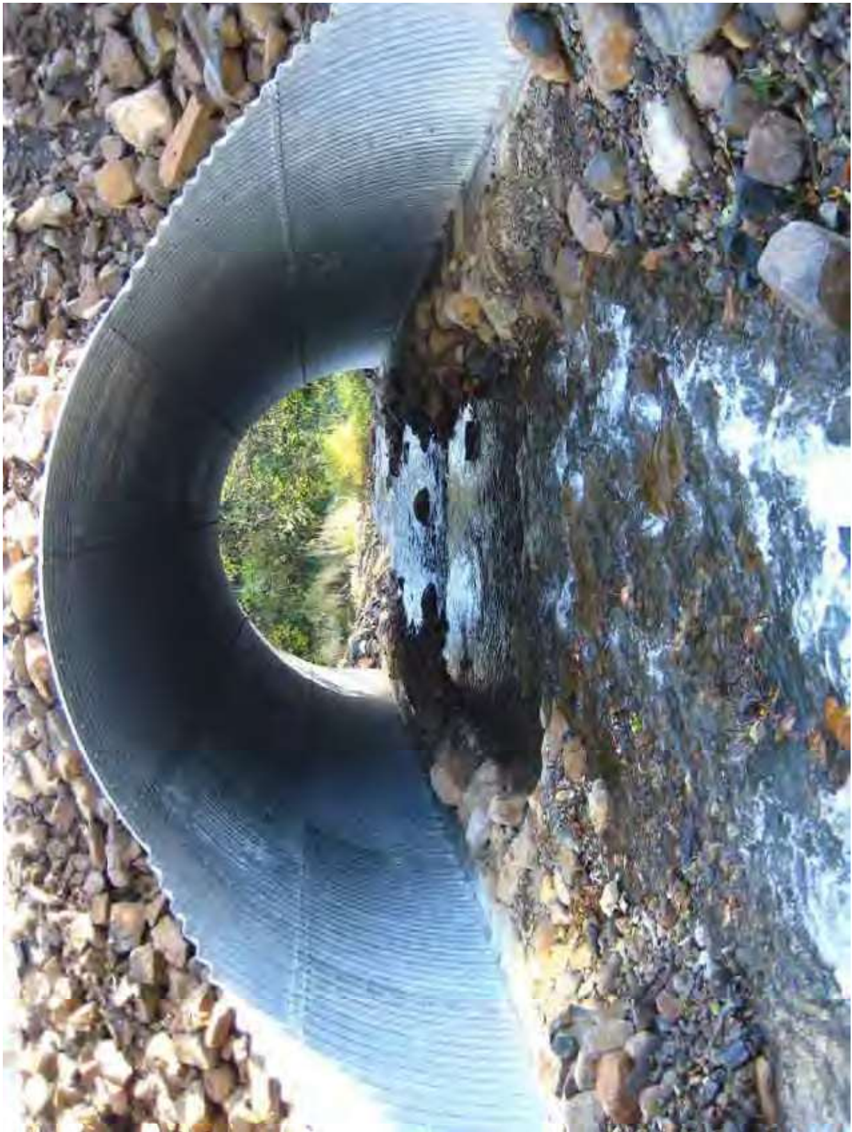
Figure 4. This arched-culvert example shows the diverse water depths and velocities, hiding and resting areas, and moist-edge habitats that support aquatic species movement.
