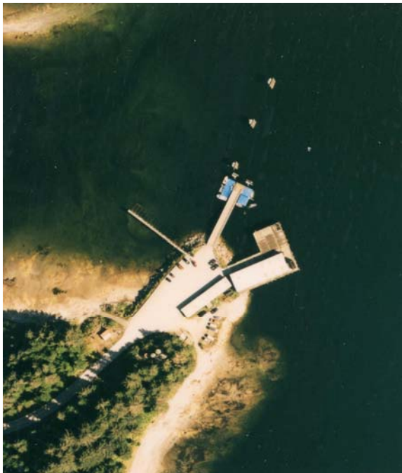
Aerial View of Ferry Terminal.
