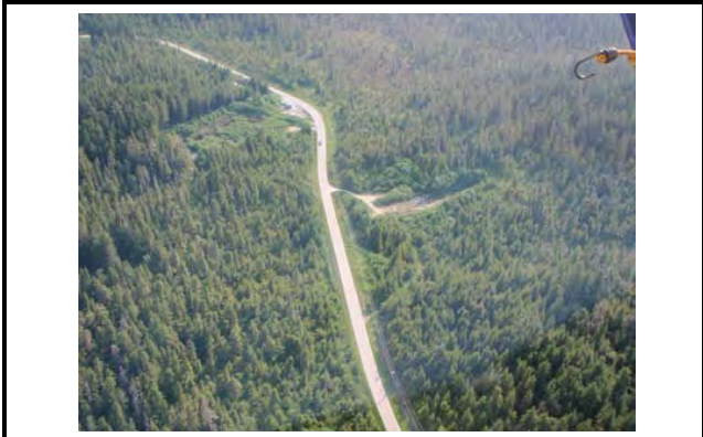
Road to Ferry Terminal and Landfill
