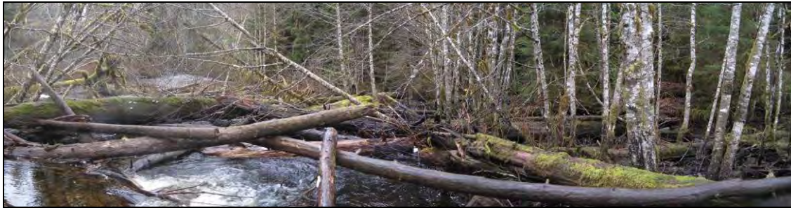
Photo 8. Complex log jam between the Access Alt. 2 and Access Alt. 3 Favorite Creek bridge crossings.
