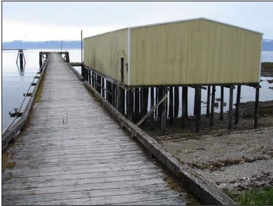
Figure 12: Fuel dock and warehouse.
