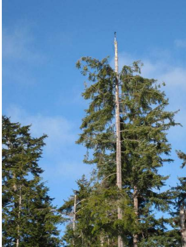
Wind meter installed at the water tower site.
