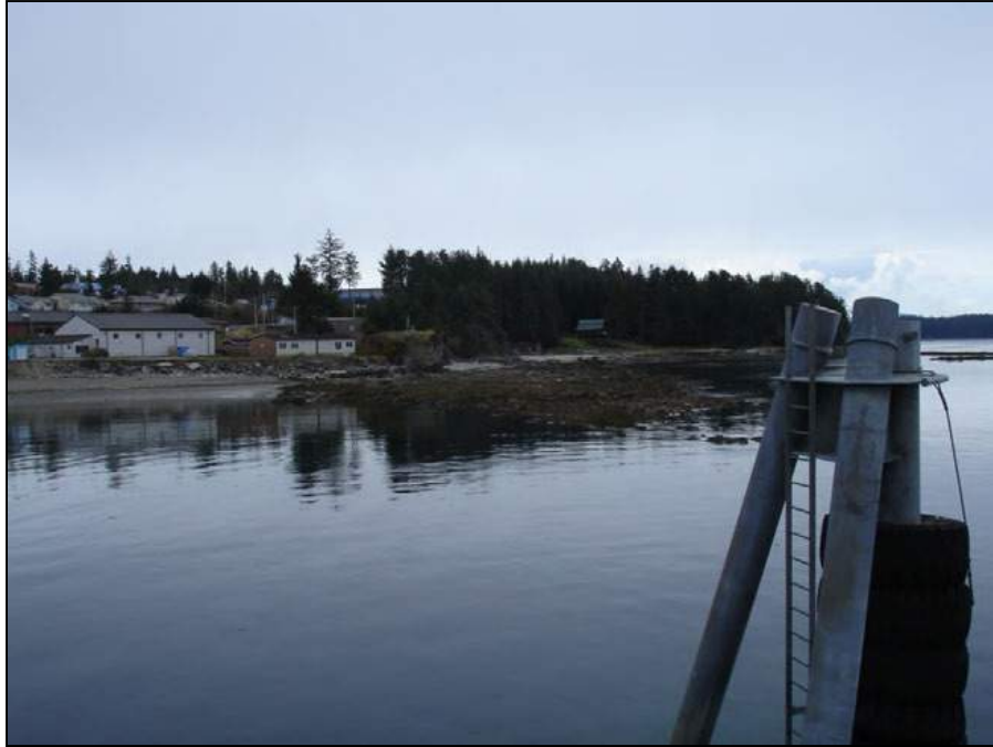
Figure 17: Dolphin at the end of the fuel dock. Fuel deliveries are made by floating a hose to the shore.
