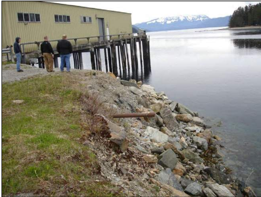
Figure 14: Looking southeast at the city dock.
