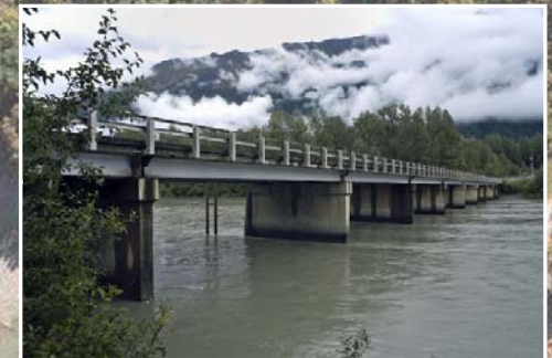
Existing Chilkat River Bridge
