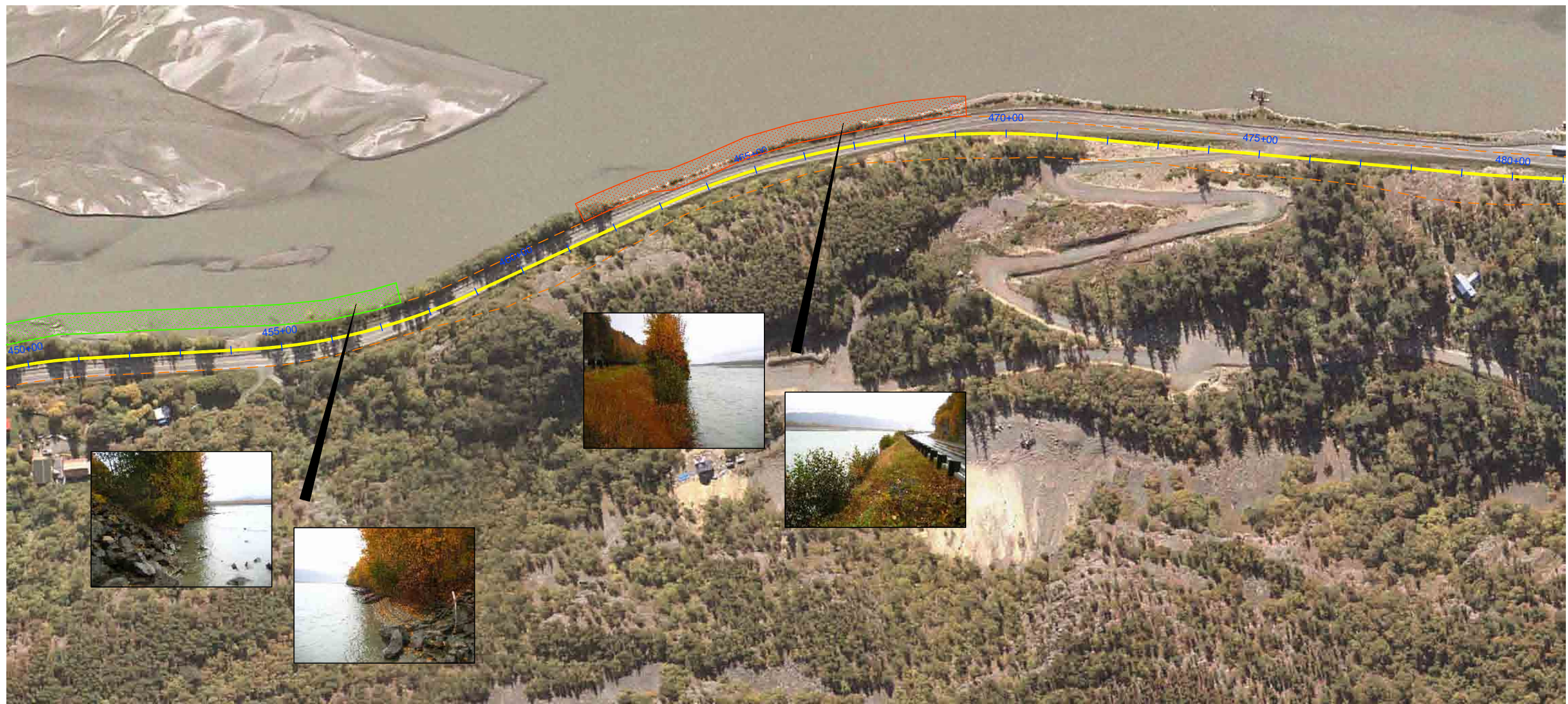
BANK STATION 444+50 TO 457+50
