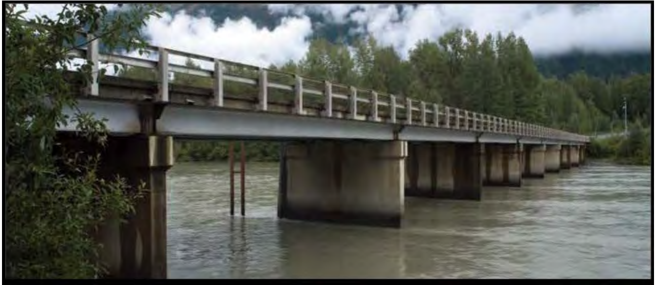
Photograph 1: Chilkat River Bridge
