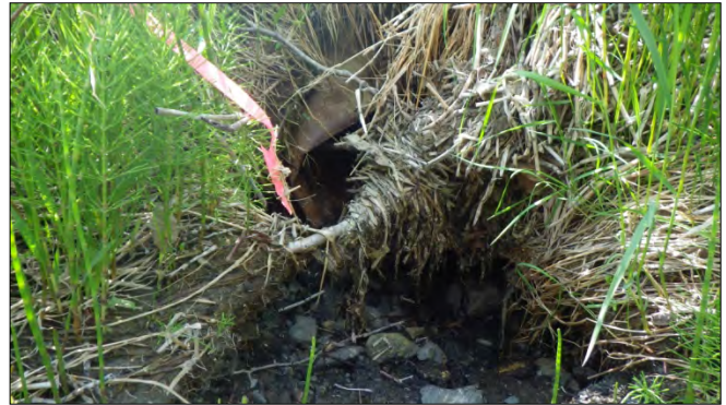
Figure 11.–HH culvert inlet (FP10).
