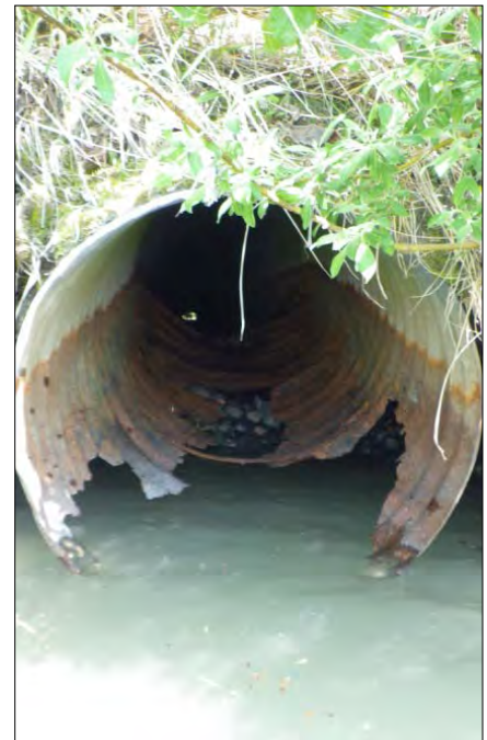
Figure 12.–HH culvert outlet (FP10).
