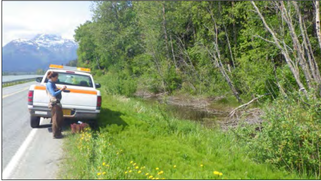
Figure 10.–Drainage upstream of HH culvert (FP10).
