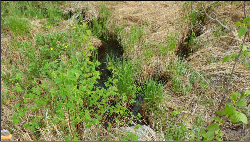
Figure 3.—Stream No. 115-32-10250-2006-3003 culvert (FP3) inlet.
