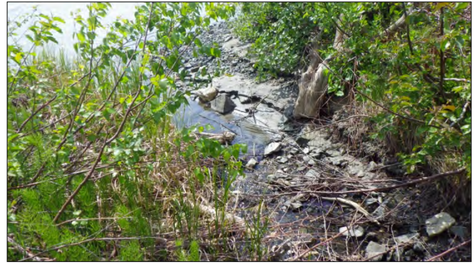
Figure 14.–Stream No. 115-32-10250-2022 downstream of HH culvert (FP11).
