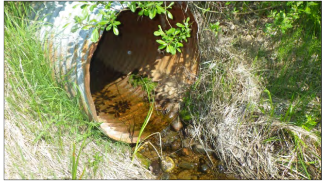
Figure 29.—MP 16.9 drainage, HH culvert outlet.
