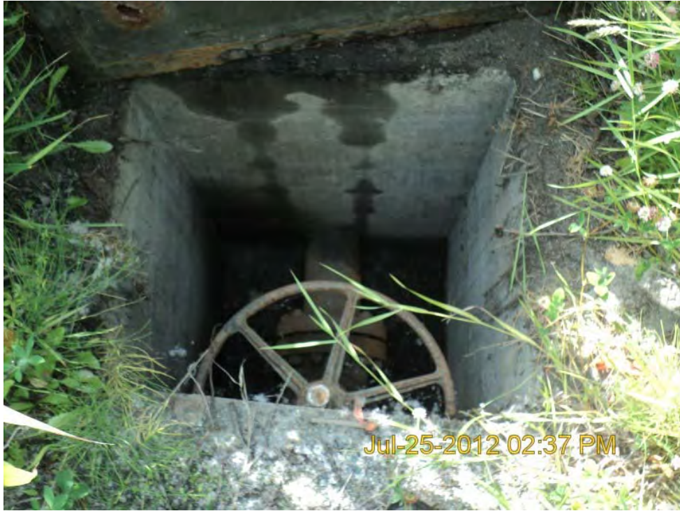
PMP 25.5 – View Inside Gate Valve 4
