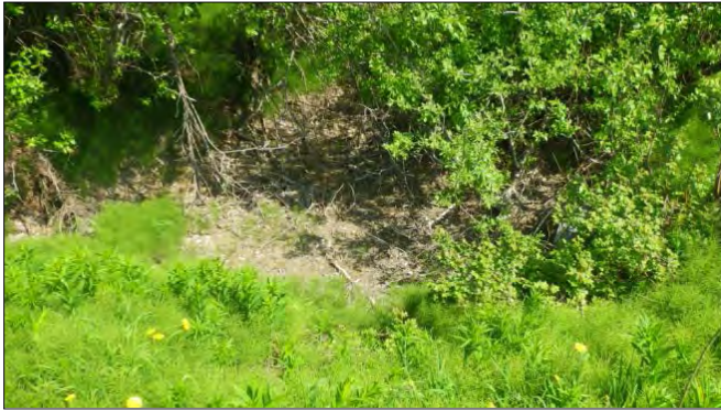
Figure 28.—MP 16.9 ditch drainage, upstream of HH.
