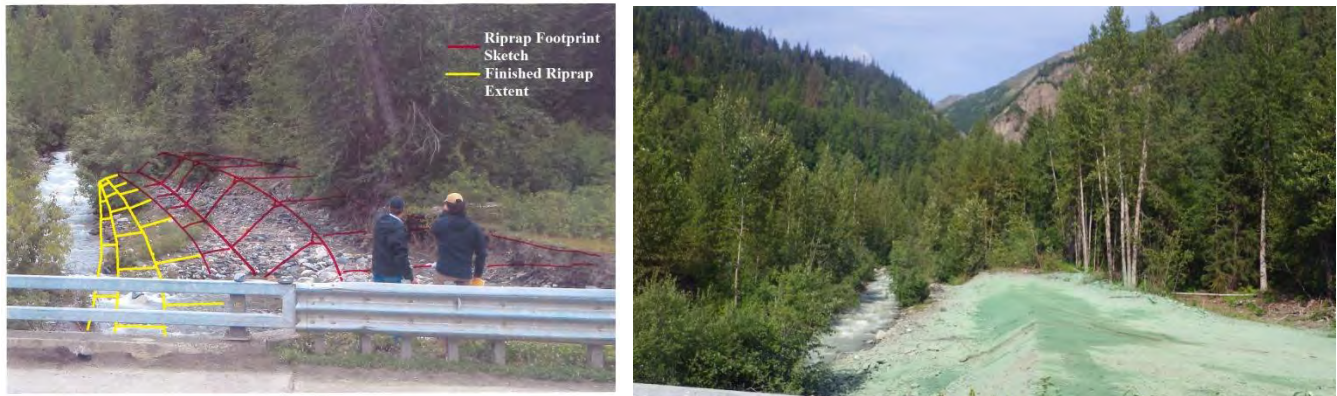
Figures 7 & 8. Left: Diagram comparing riprap plans and finished extent of riprap placed. Right: Finished bank stabilization after recent hydroseeding. Note the clump of trees in the bottom left corner of the photos gives a reference to compare the sketch and final work (August 5, 2013).
