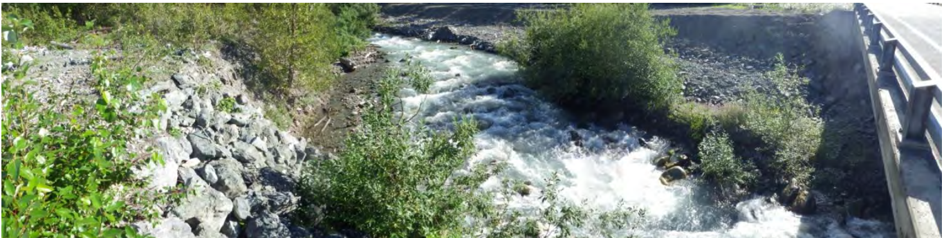
Figure 5. Little Boulder Creek view upstream of bridge following repair work (August 5, 2013).
