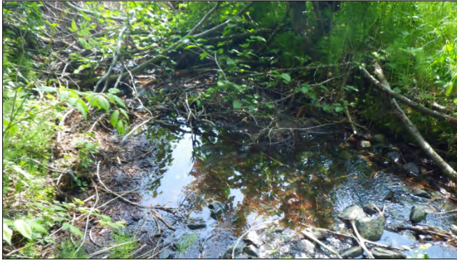
Figure 13.–Stream No. 115-32-10250-2022 upstream of HH culvert (FP11).
