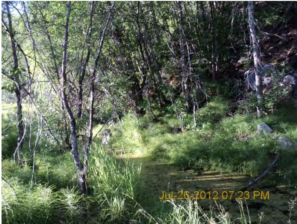
PMP 17.7 – Pipeline Trench on East Side of Haines Highway (Photo Taken from Pipeline Mound – Looking North)
