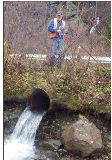
Figure 23.—Bob Trousil (ADOT&PF) at the 12 Mile Creek HH culvert (FP17) outfall, waterfall in background (dated October 24, 2013, courtesy of Matt Kern).
