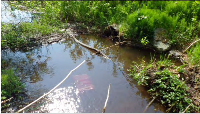
Figure 7.–HH culvert (FP7) inlet pond.
