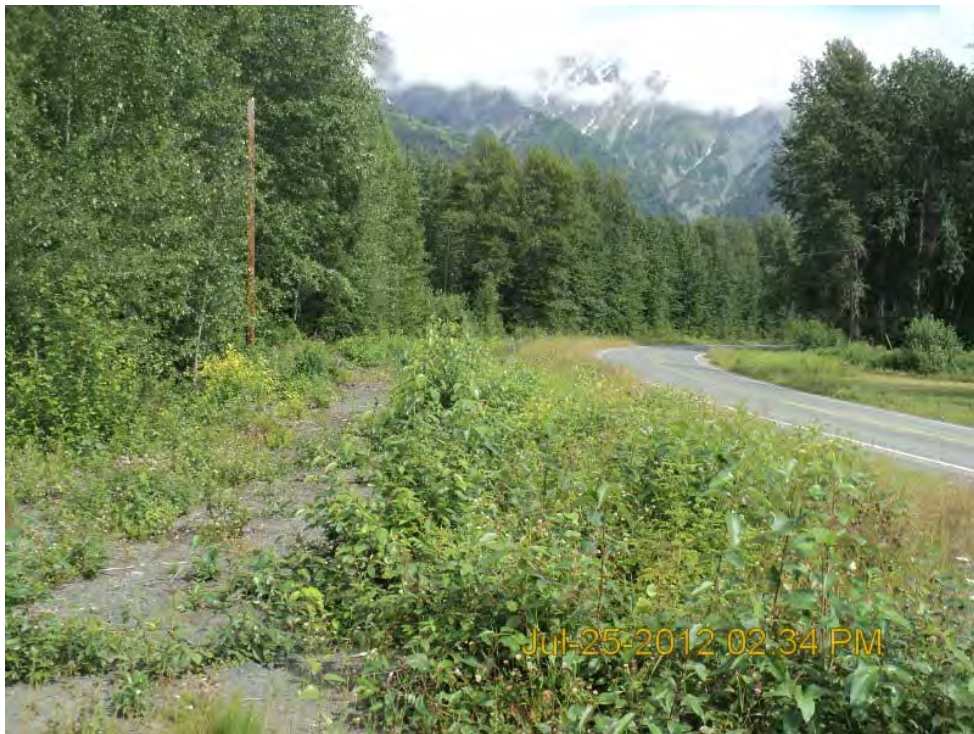
PMP 25.5 - East of GV4 on North Side of Haines Highway (Looking East)
