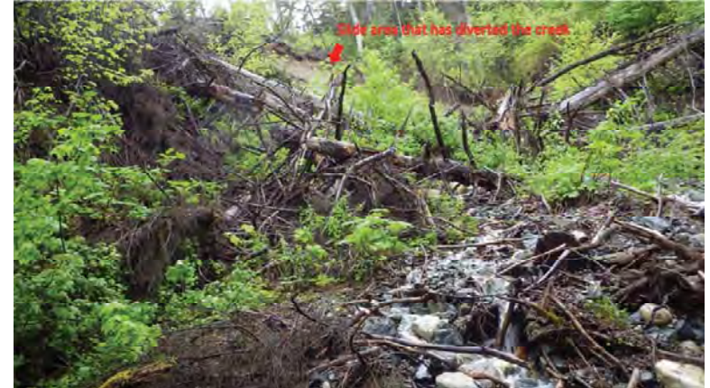
Figure 4. Looking upstream above the highway at stream no. 115-32-10250-2016-3020 headwaters and a landslide. The arrow shows where the slide occurred that diverted the creek.
