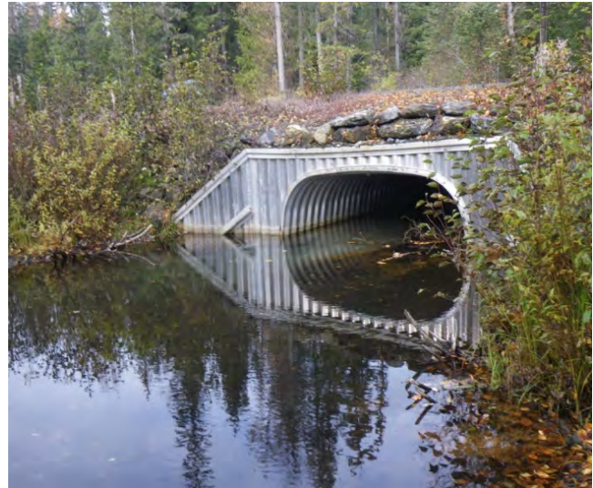
Figure 35.–Culvert CV-12 outlet.
