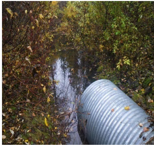
Figure 27.–Culvert CV-8 outlet.
