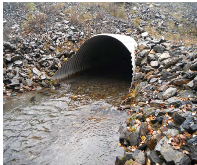
Figure 29.–Culvert CV-9 outlet.
