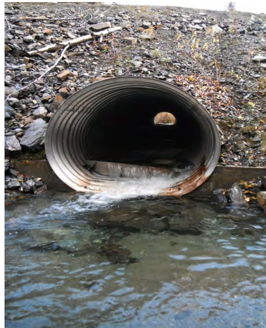
Figure 37.–Culvert CV-13 outlet.
