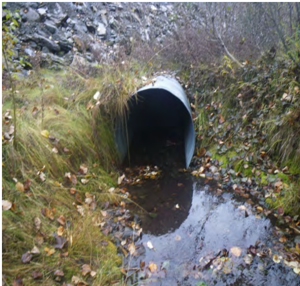
Figure 26.–Culvert CV-8 inlet.
