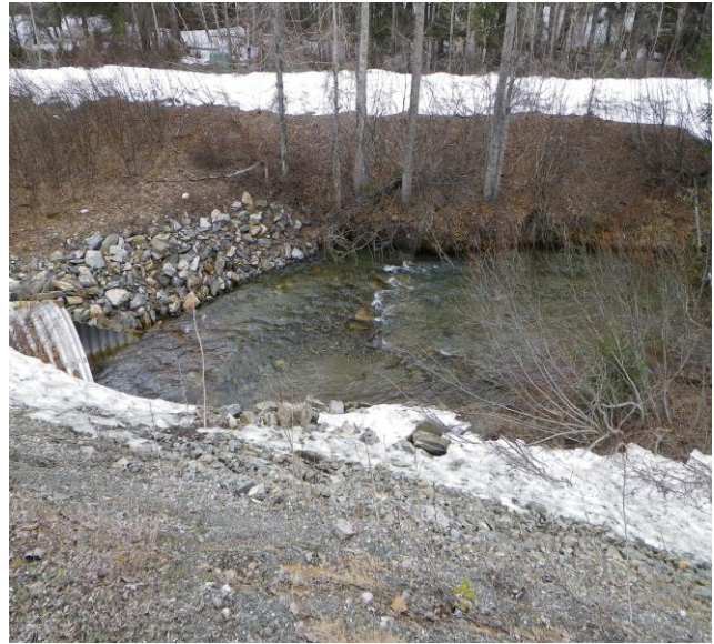
Figure 7.—Culvert CV-9 outlet 5/10/12.
