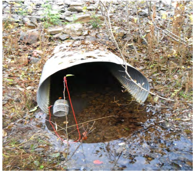
Figure 31.–Culvert CV-10 outlet.
