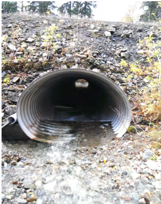
Figure 36.–Culvert CV-13 inlet.
