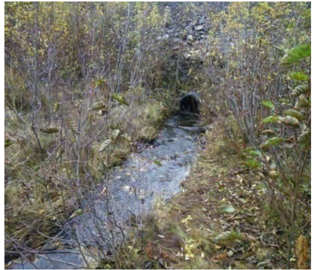
Figure 9.—Culvert draining WT-6.
