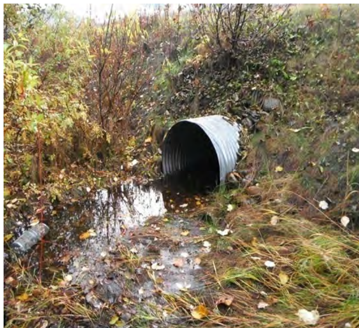
Figure 20.—Inlet to culvert CV-6.
