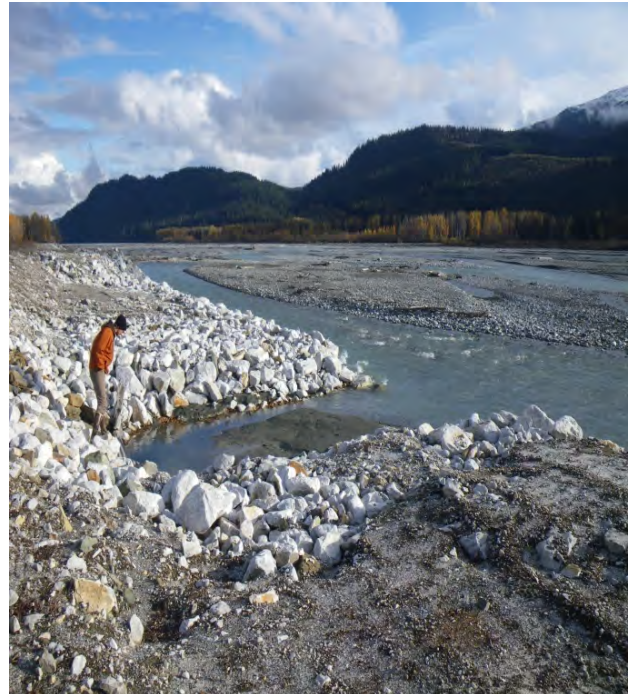
Figure 22.—Fill material placed near CV-6.
