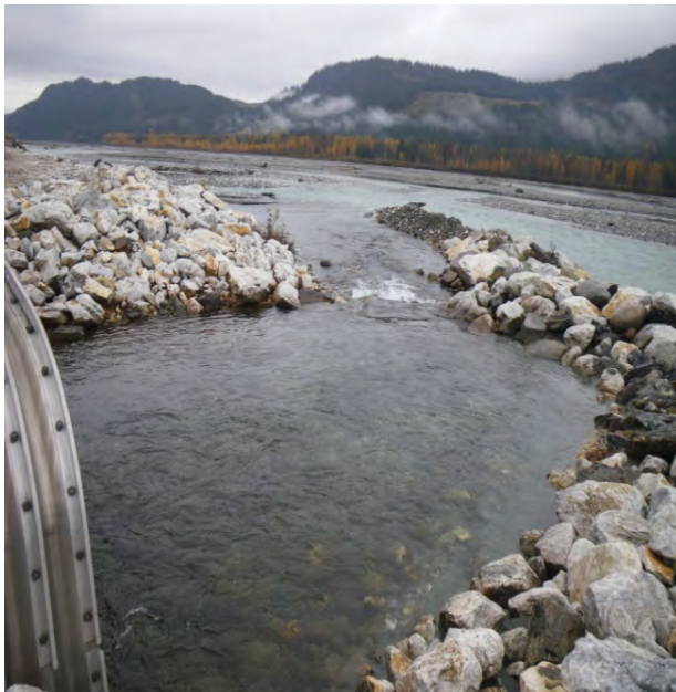
Figure 24.—Outlet pool and fill material near CV-7.
