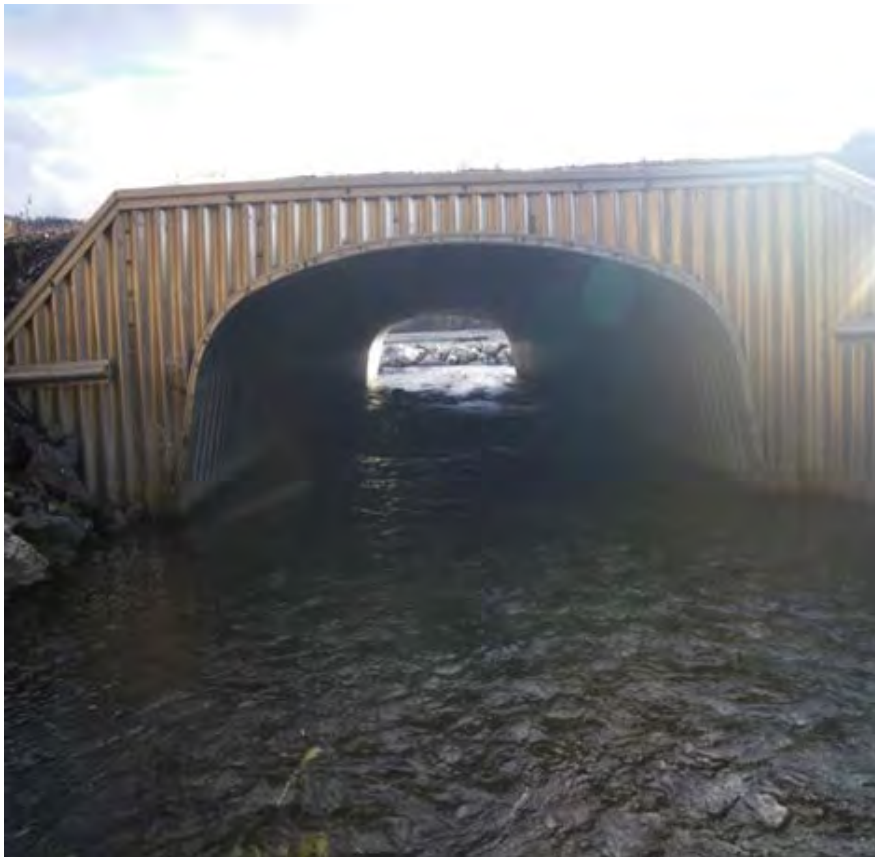
Figure 23.—Inlet to culvert CV-7.
