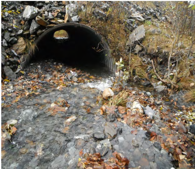
Figure 32.—Culvert CV-11 inlet.
