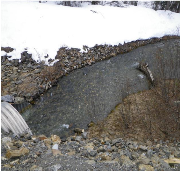
Figure 6.—Culvert CV-9 inlet 5/10/12.
