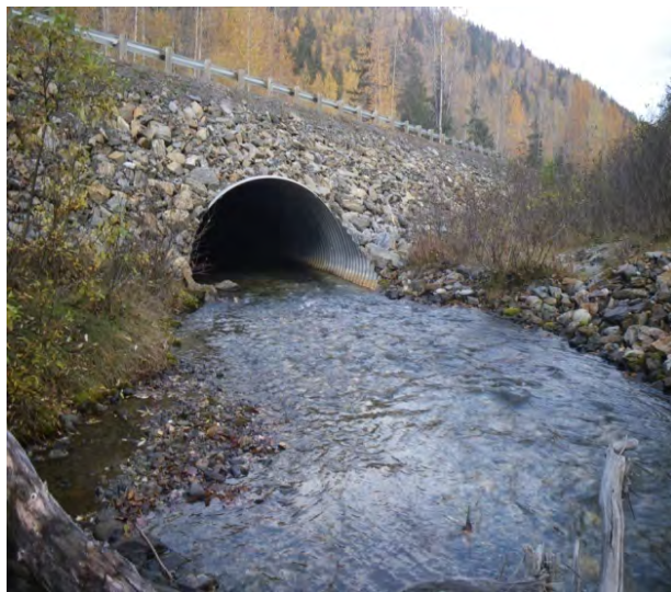
Figure 28.–Culvert CV-9 inlet.
