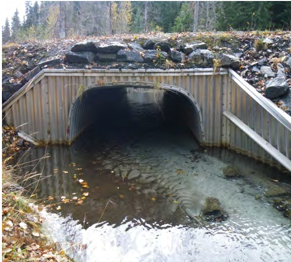
Figure 34.–Culvert CV-12 inlet.
