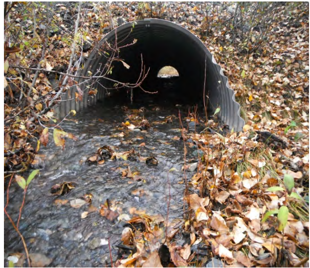
Figure 33.—Culvert CV-11 outlet.
