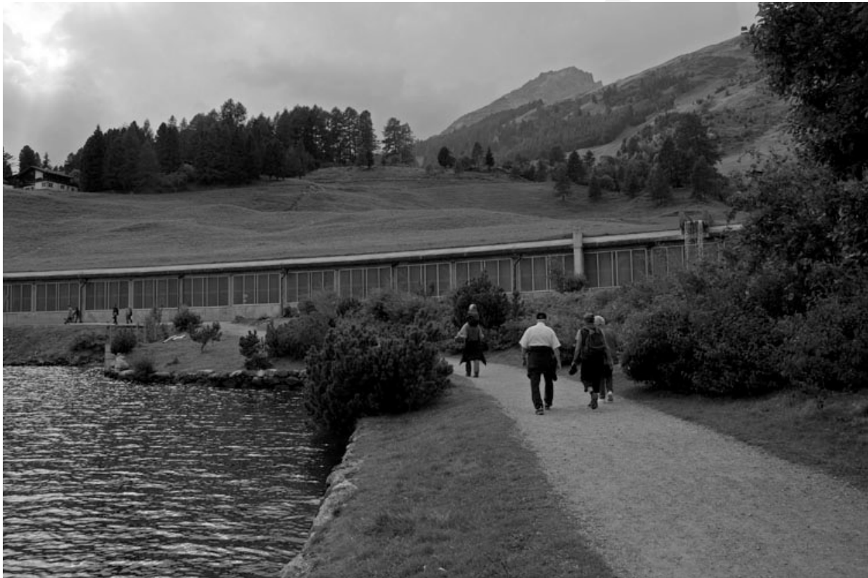
Figure 15: Shed-roof Gallery Snowshed, Davos, Switzerland
