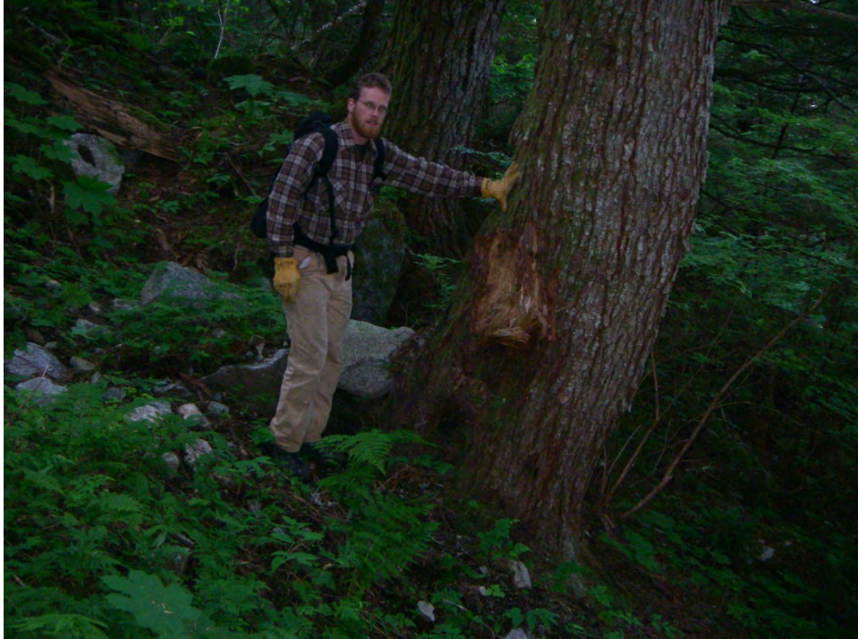
RF31. View south/down alignment at rockfall with freshly gouged trees.
