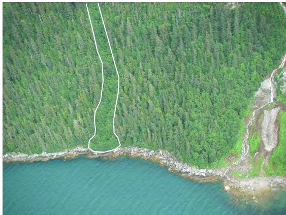
DF30. Disturbed vegetation marks path of debris flow.
