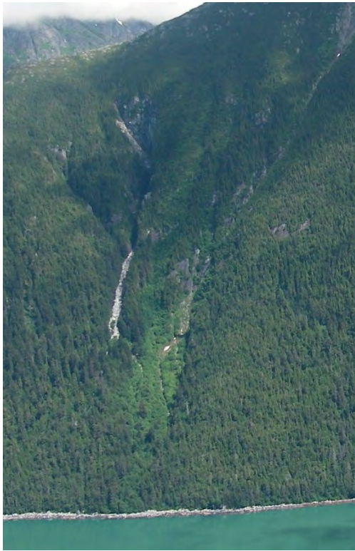
RF19. View east/upslope at large rockfall area.
