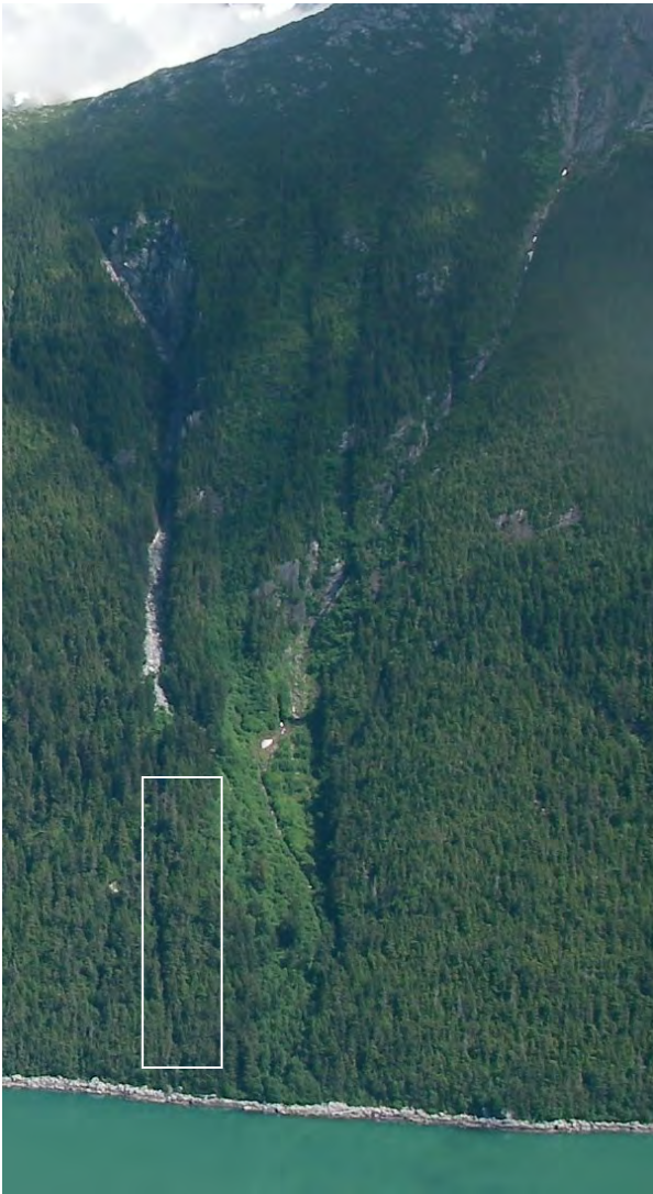
RF20. View east/upslope at rockfall area and avalanche path.
