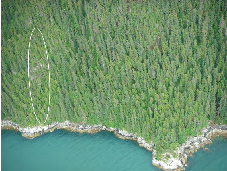
RF36. View east/upslope at rockfall hazard.
