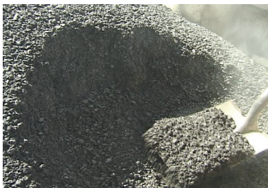
Asphalt mixture in a haul unit
