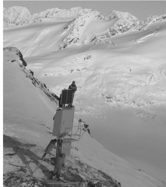
Figure 8- Avalanche Guard Installation
