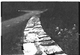
Top: crash tested and approved concrete-core barrier wall under construction. Bottom: completed concrete-core barrier wall.
